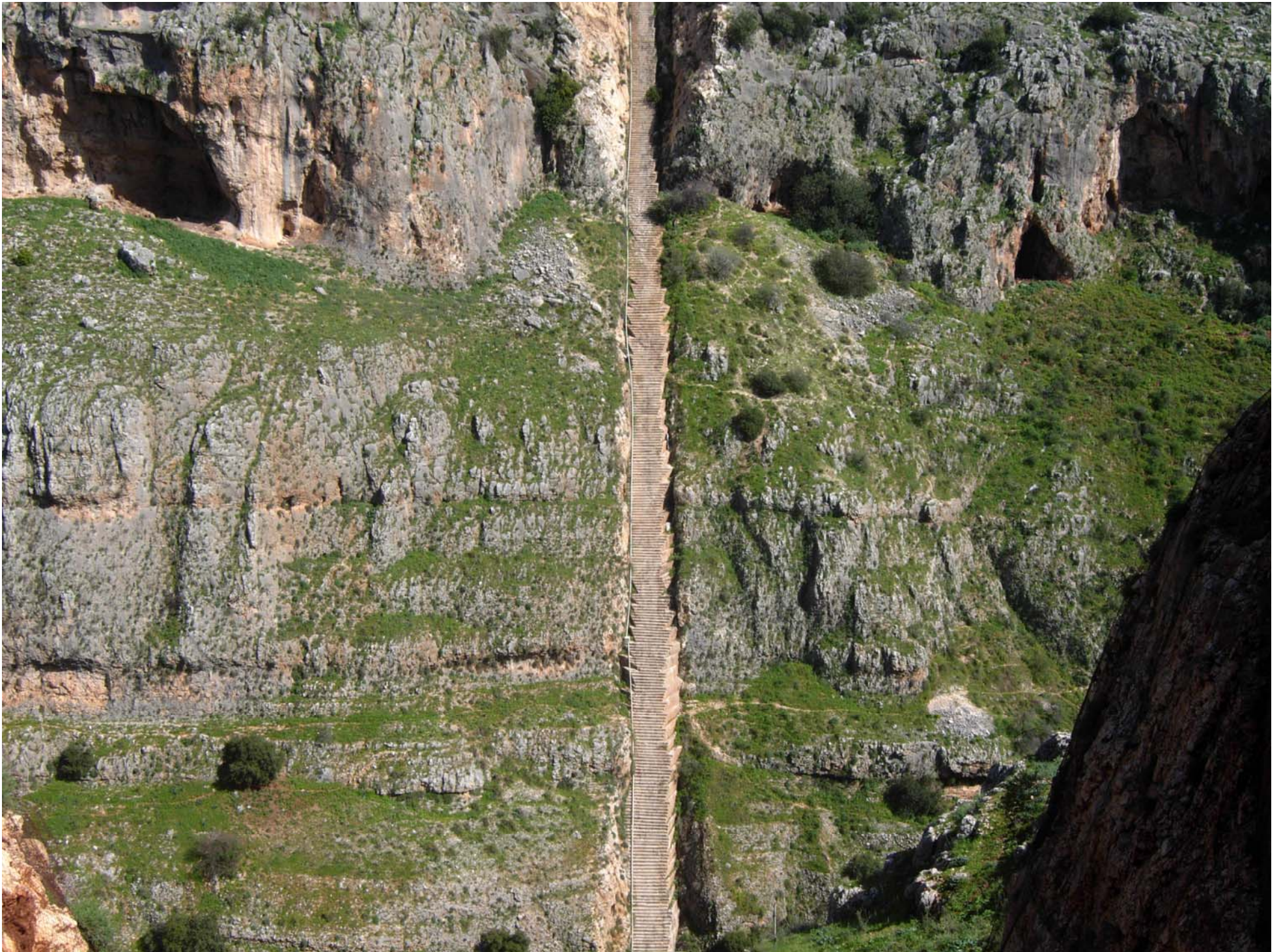
Inverted siphon of the national water carrier - Israel
