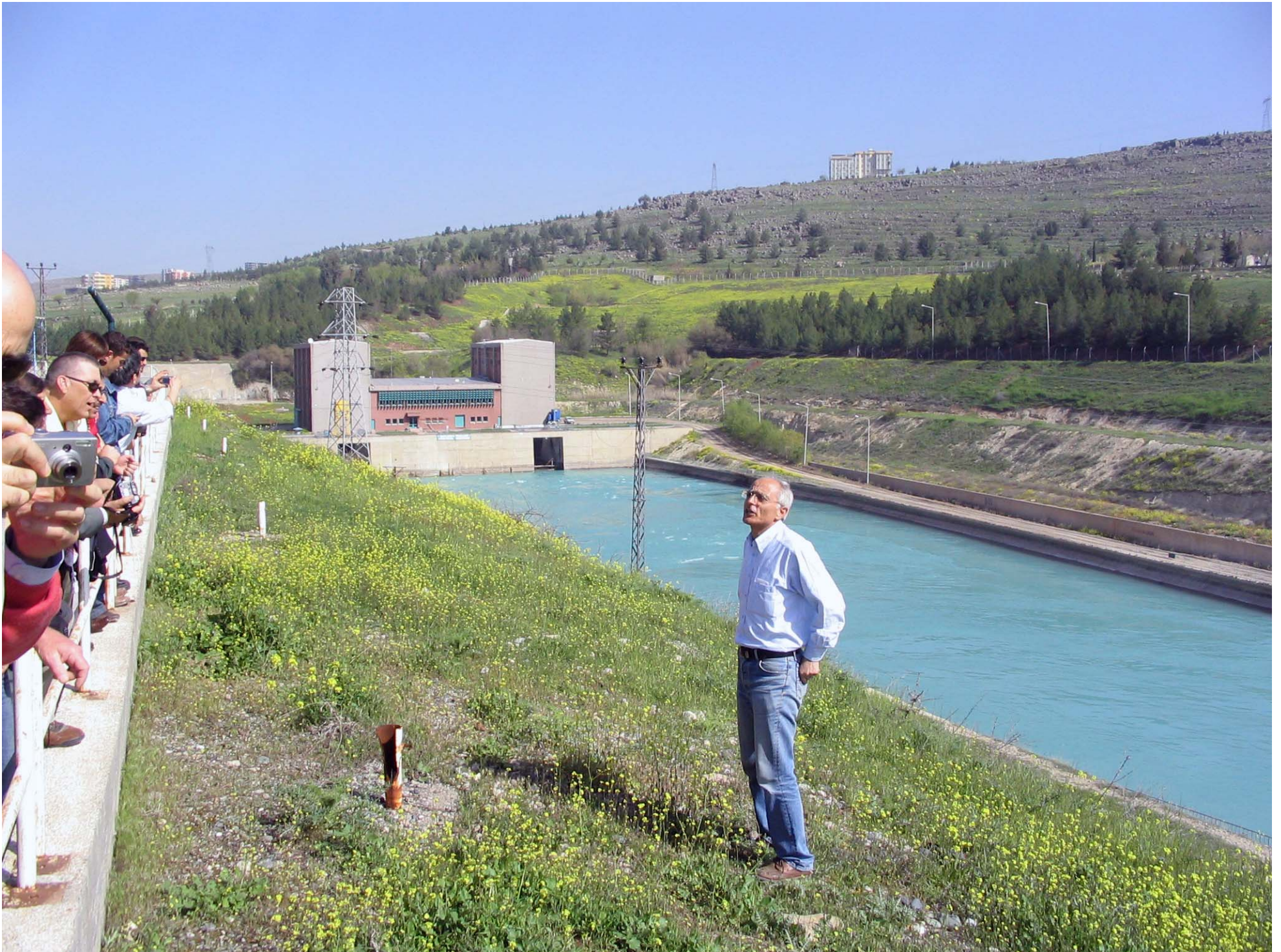
Sanliurfa Irrigation Tunnels - South-East Anatolia, Turkey Each tunnel is 26.4 km long - The total flow rate is 328 qm/s
